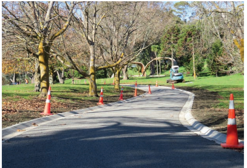
Contractors put finishing touches to the road sealing.
